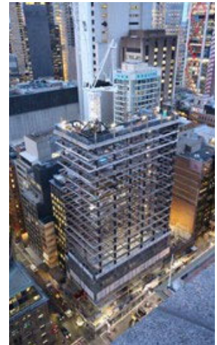
20 Martin Place stripped back to its steel frame. Photo: Built
