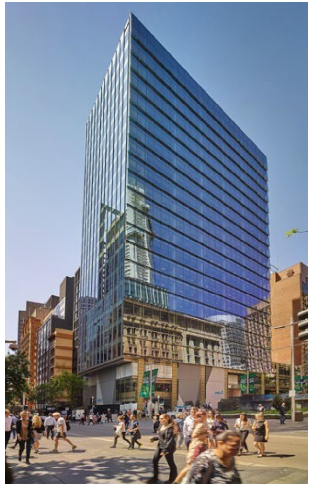
20 Martin Place transformed through circular design. Photo: Built
